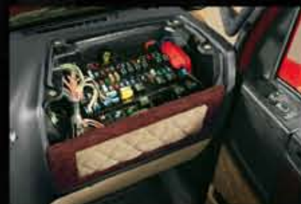
Power Distribution Module (PDM)
